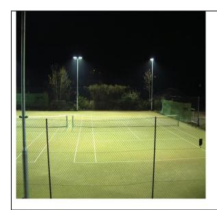
Corner lit layout - typically 10m with 'Projector' fitting. (Min. column height 8m)
