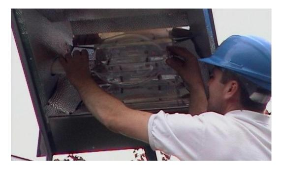
Maintenance of the lighting system is one of the most important issues to consider when choosing equipment. Apart from replacing lamps, the lens and reflector of each fitting have to be kept clean and the aiming of the fitting may need to be adjusted to retain uniformity.
