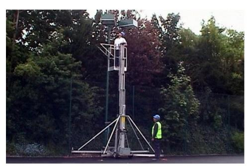
Health and safety requirements should be taken into account when servicing floodlighting. Adequate protection of the court surface must be considered with the use of a high level maintenance vehicle or working platform.
