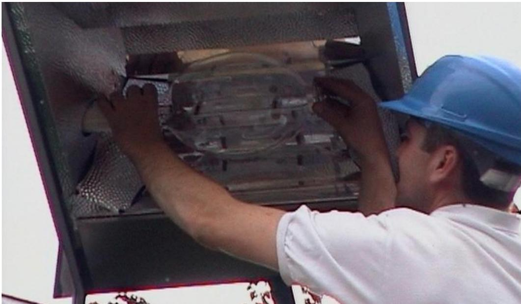
Maintenance of the lighting system is one of the most important issues to consider when choosing equipment. Apart from replacing lamps, the lens and reflector of each fitting have to be kept clean and the aiming of the fitting may need to be adjusted to retain uniformity.
