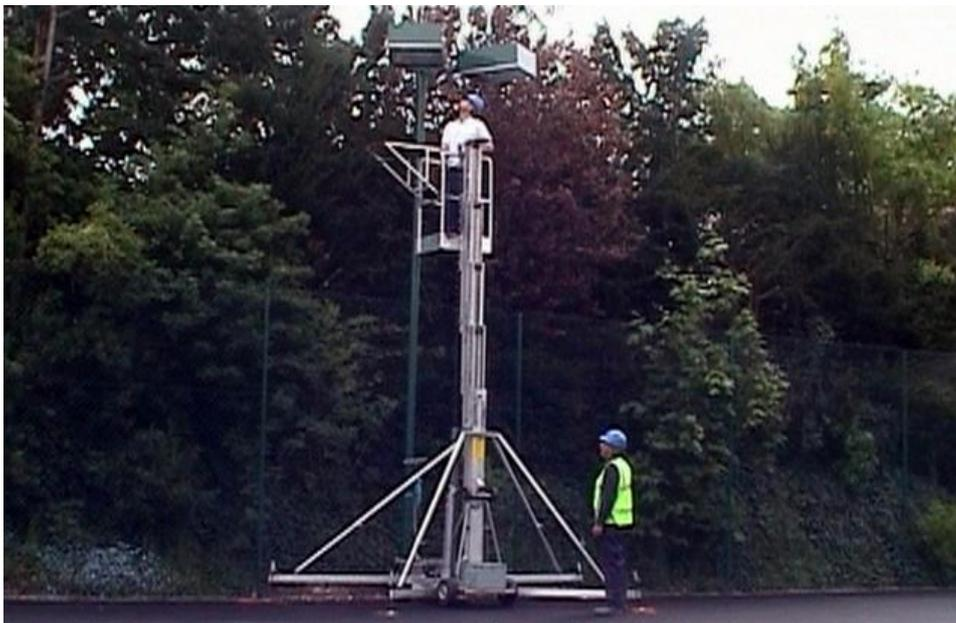
Health and safety requirements should be taken into account when servicing floodlighting. Adequate protection of the court surface must be considered with the use of a high level maintenance vehicle or working platform.
